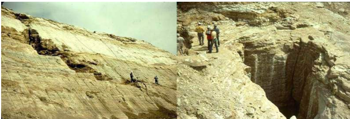
Figure 3-12 Solution features exposed during earthworks for the Clarence Cannon Dam, central Missouri. Courtesy of J. Higgins, Colorado School of Mines.
